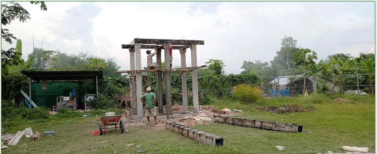
[The progress of installing the water tank]
